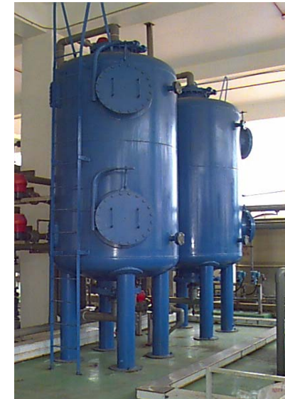
The full scale ion exchange system for Ag removal, Capacity=40M 3 /Hr
