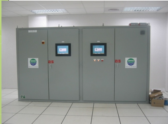
PLC control panel
