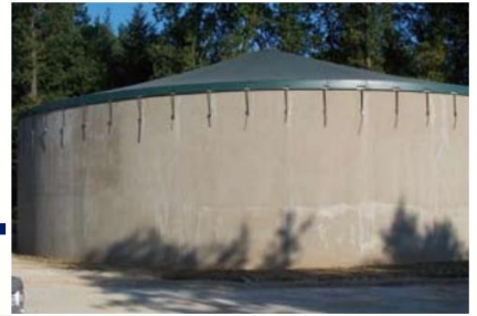
Photo 5: Covered digestate storage tank
