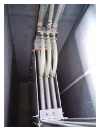
Submerge MF membrane Cassette
